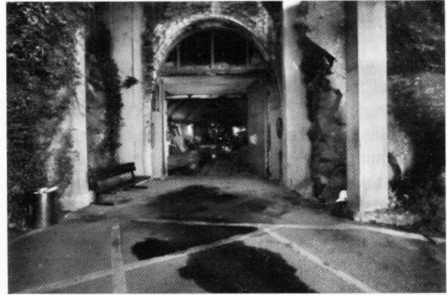
Entrance portal to the 1898 railway tunnel at St Aubin, later adapted by the Germans as Ho5. The tunnel, part of which is now a depot for bicycle hire, was converted to metre gauge by the occupiers – a section of this track is visible.
